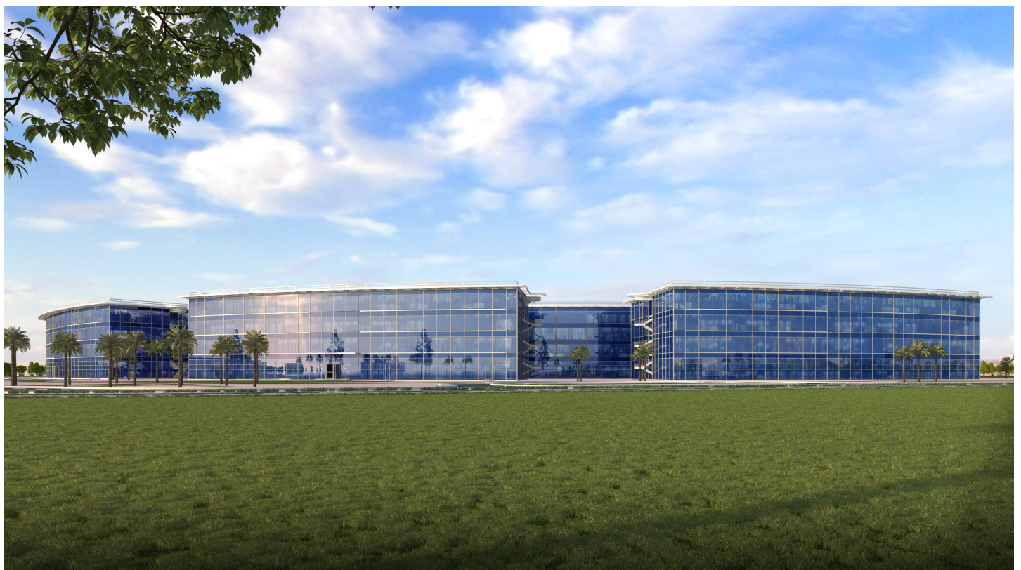
Etisalat Misr New Premises at Smart Village
