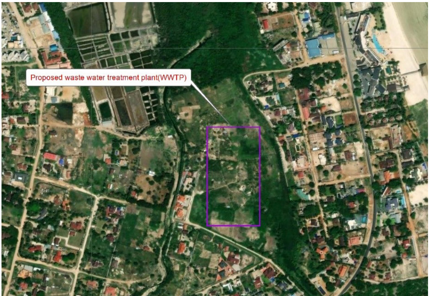
Wastewater Treatment Plant in Mbezi
