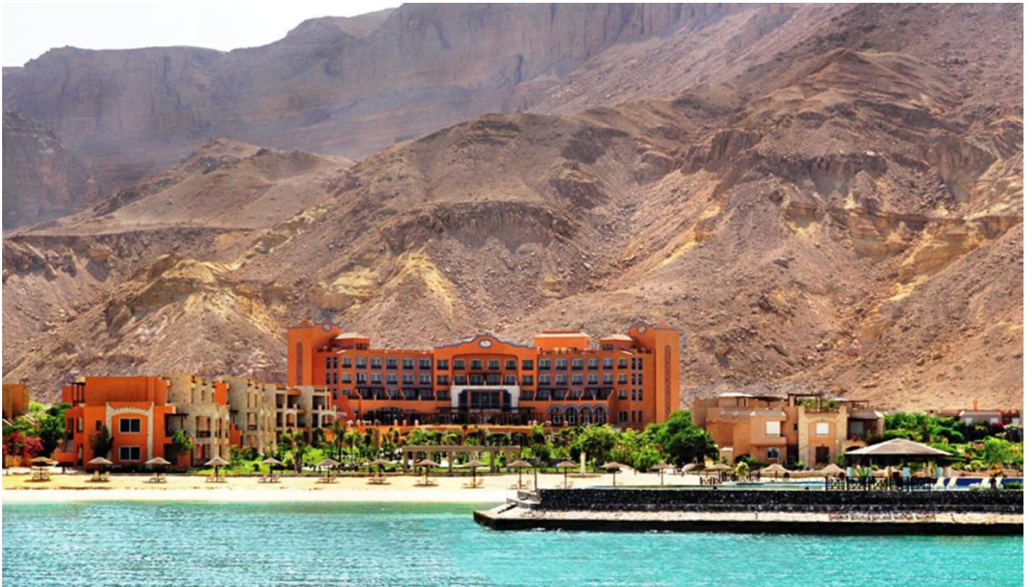
Renovation of Movenpick Al-Ain Al-Shokhna
