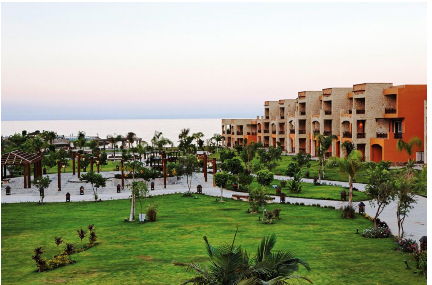
Renovation of Movenpick Al-Ain Al-Shokhna
