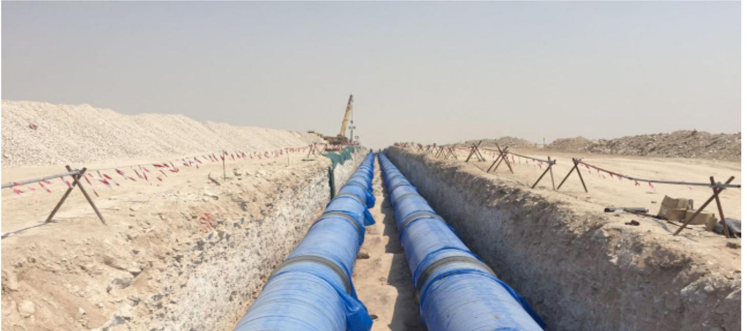
This project involves the design of ductile iron pipelines (approximately 71 km long) ranging from 600 mm to 1,600 mm in diameter. The desalinated water transmission pipeline is expected to be completed ahead of the QEZ3 desalination plant.
