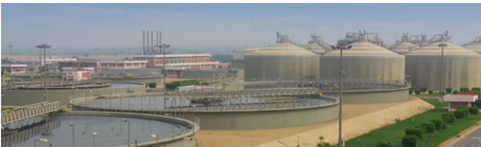
El-Gabal El-Asfar WasteWater Treatment Plant (Stage II - Phase II), Egypt
