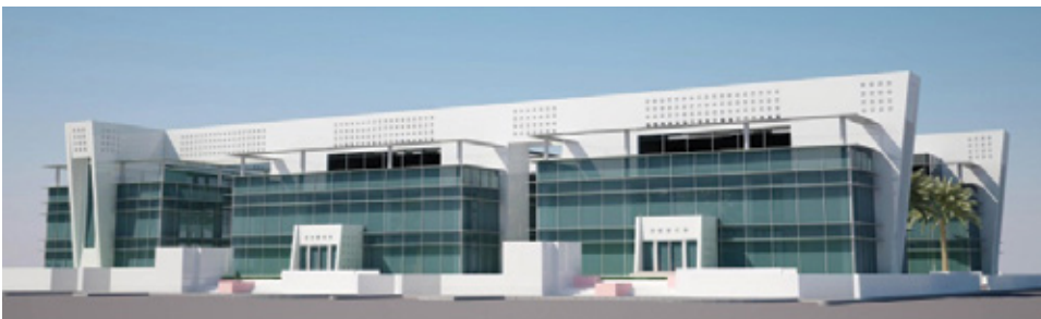
Arabian Gulf Holding Co. Office Building, Kuwait
